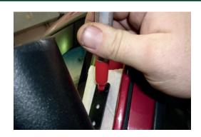
12. Apply silicone sealant to holes and insert mounting plugs.
