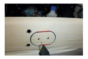
7. Drill mounting holes to 16mm.
